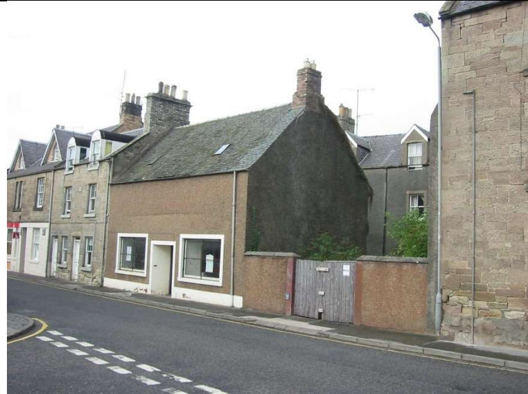
20-24 South Street in May 2007, before purchase.
